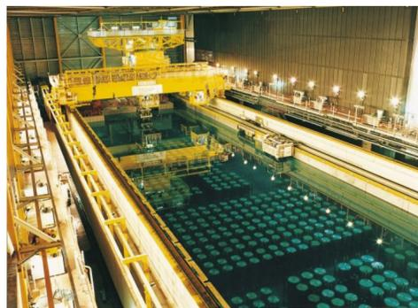
Fig. 2: Storage pond for used fuel at the Thermal Oxide Reprocessing Plant at the UK's Sellafield site (Sellafield Ltd)
